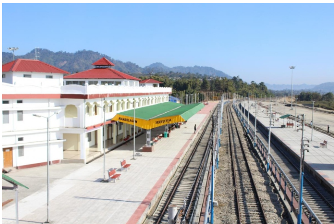
Naharlagun Railway Station
